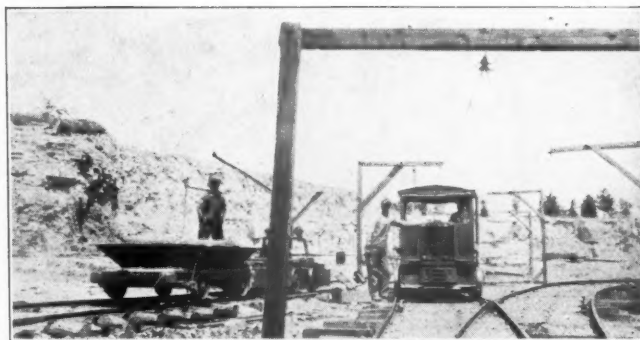
Electric and Gasoline Trucks in Yard
